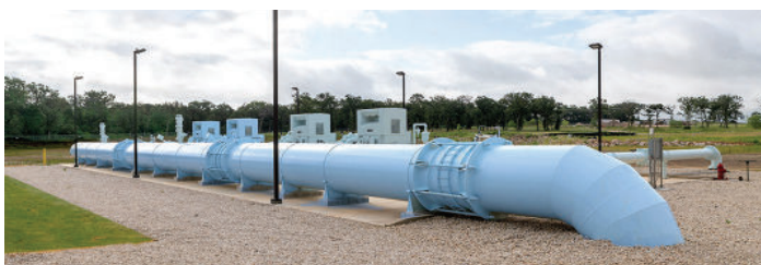
Vista Ridge Water Supply Project, TX
