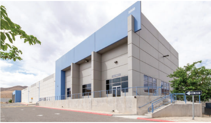
3200 USA Parkway, which CapRock Partners recently acquired in Reno, Nev.
