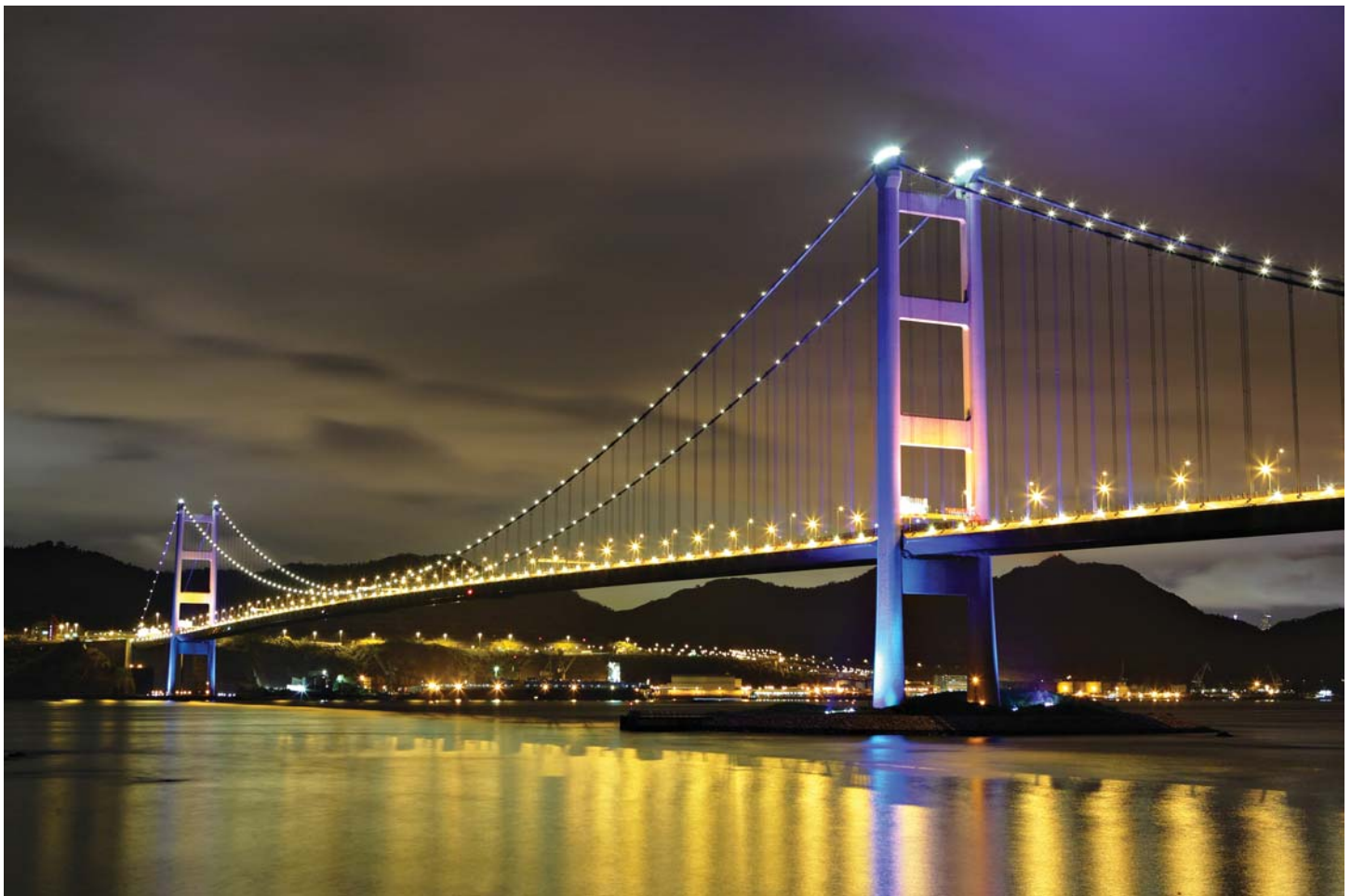
TSING MA BRIDGE HONG KONG
